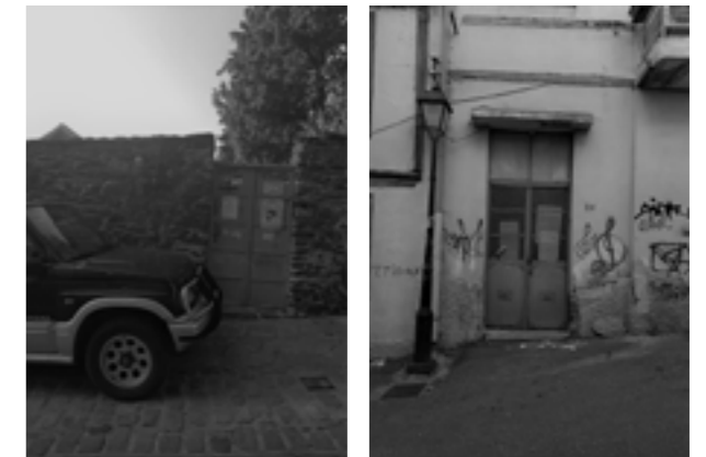
Fig.12, 13: Public space used as a parking area.
